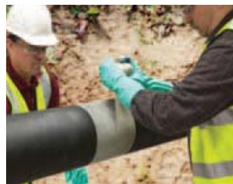
Tightly wrap repair area
