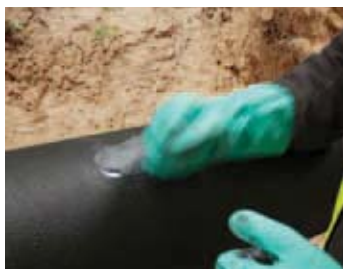
Mix and apply epoxy putty
